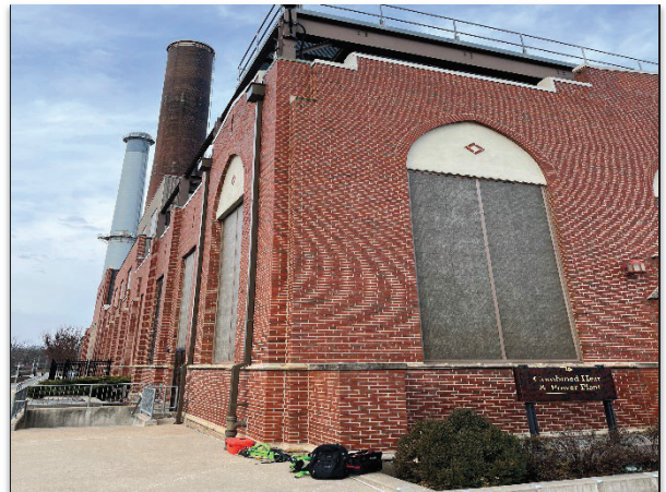
Figure (2) – SE Corner of Building 1923.
