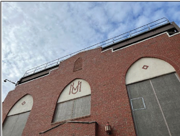
Figure (3) – Elevated terra cotta/plaster features on Building 1923.
